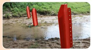
**6.** To re-position, the flood posts can be quickly and easily positioned back into place and the wires re-tensioned as shown above.
