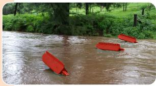
3. The flood posts have held the wires above the water line in this example.
